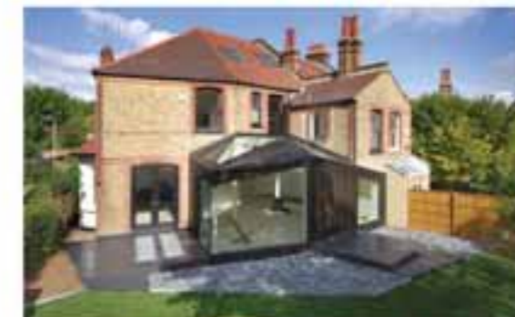
Park Avenue South
