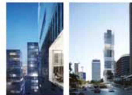
486 Mina El Hosn Housing, Offices, Retail Area
